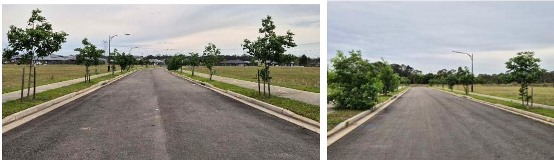
Figures 10 & 11: The appearance of the existing site condition can be observed. (Source: Oates 7/11/2024).
