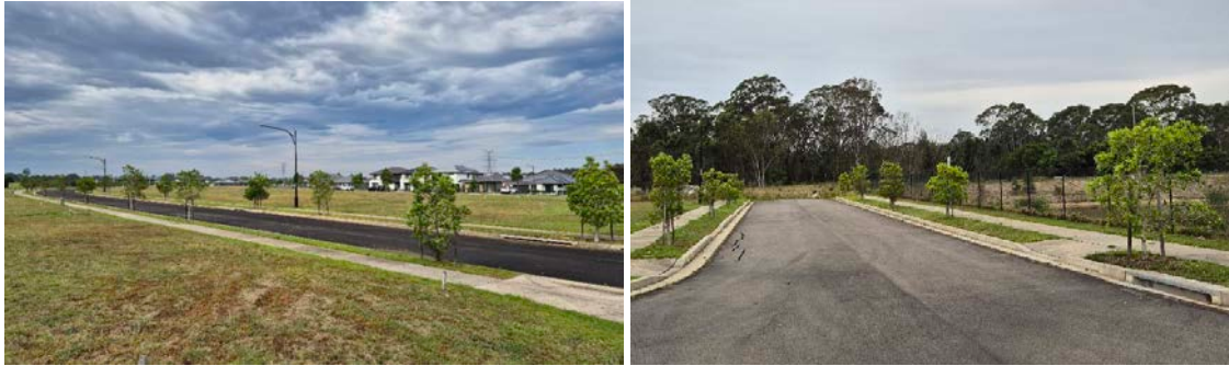
Figures 6 & 7: The appearance of the existing site condition can be observed. (Source: Oates 7/11/2024).
